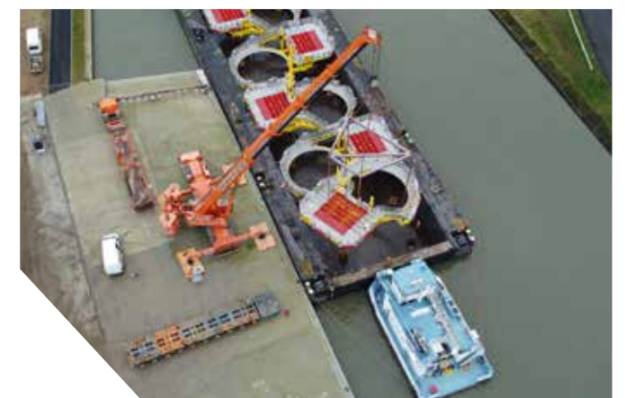
Load-out of the platforms at Willems
